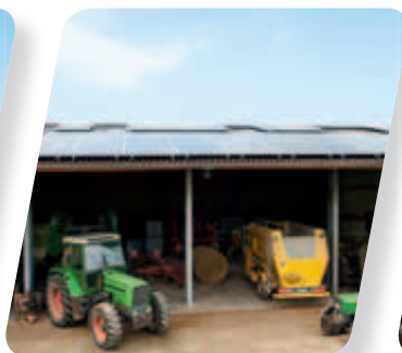
Friolzheim, Germany: Farm with Suntech modules
