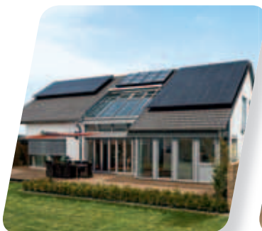
Öschelbronn, Germany: House with Suntech modules
